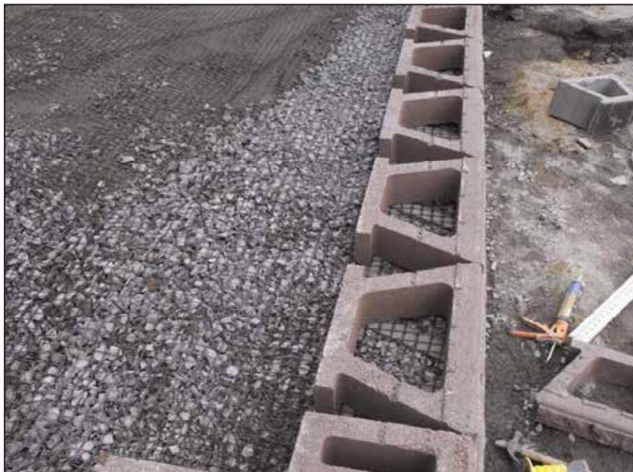
Drainage Aggregate (Inside and behind units)
