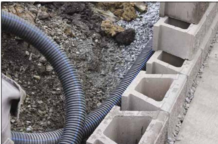
Drainage Pipe Placement
